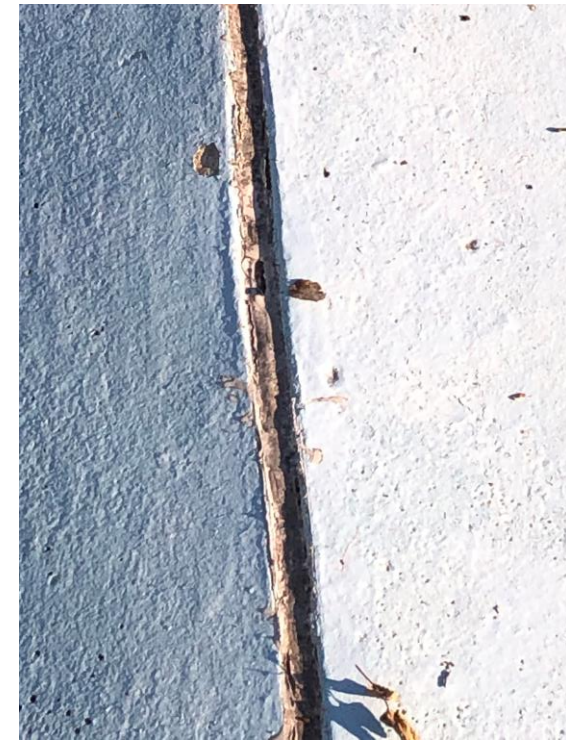
Expansion joint erosion
