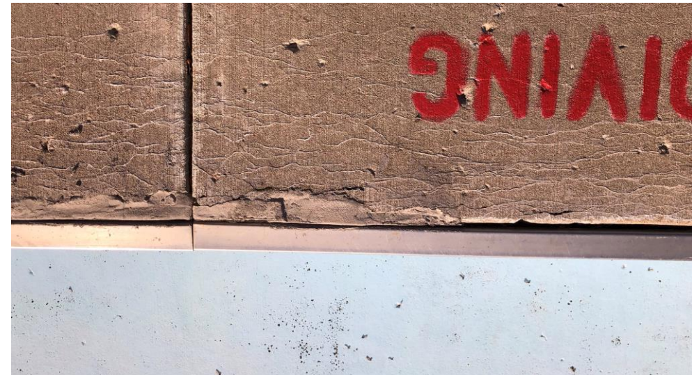
Concrete deck erosion
