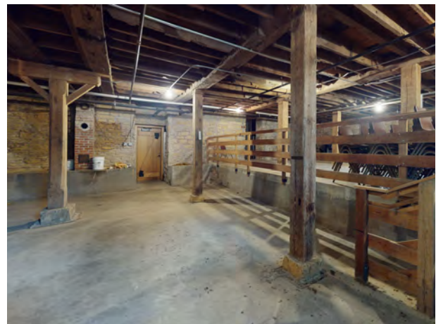
Lower level, concrete floor.
