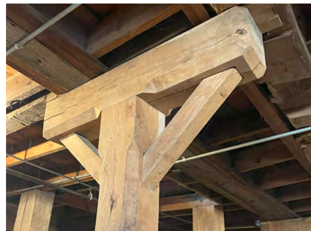
Typical detail supporting the first floor.
