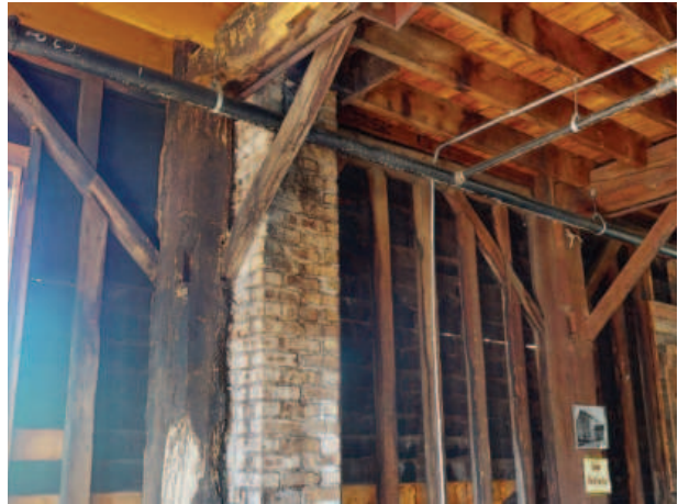
Second floor, missing bent members.
