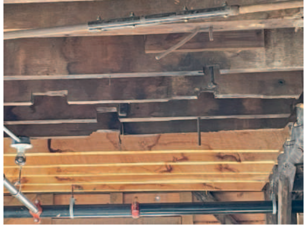
Compromised wood members supporting first floor.
